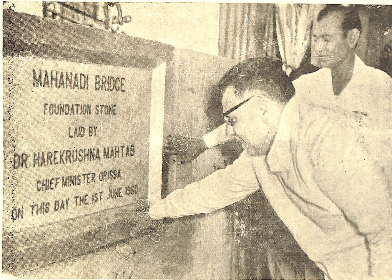
Chief Minister, Dr. Harekrushna Mahtab. laying the foundation stone of the bridge over the Mahanadi
