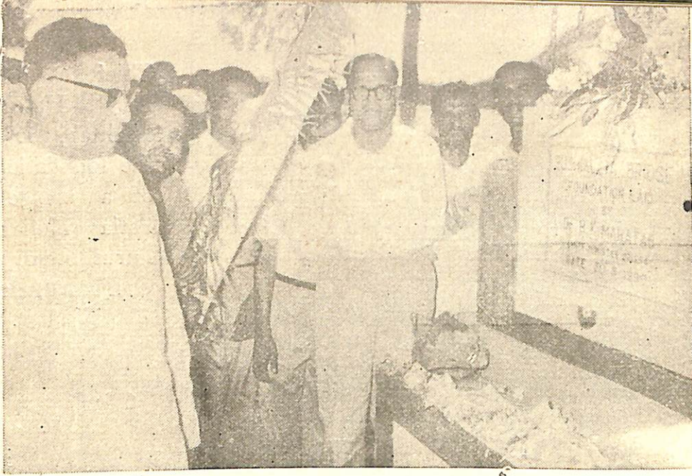
Chief Minister, Dr. Harekrushna Mahtab laying the foundation Stone of a bridge over the Rushikulya river near Purushottampur in Ganjam district
