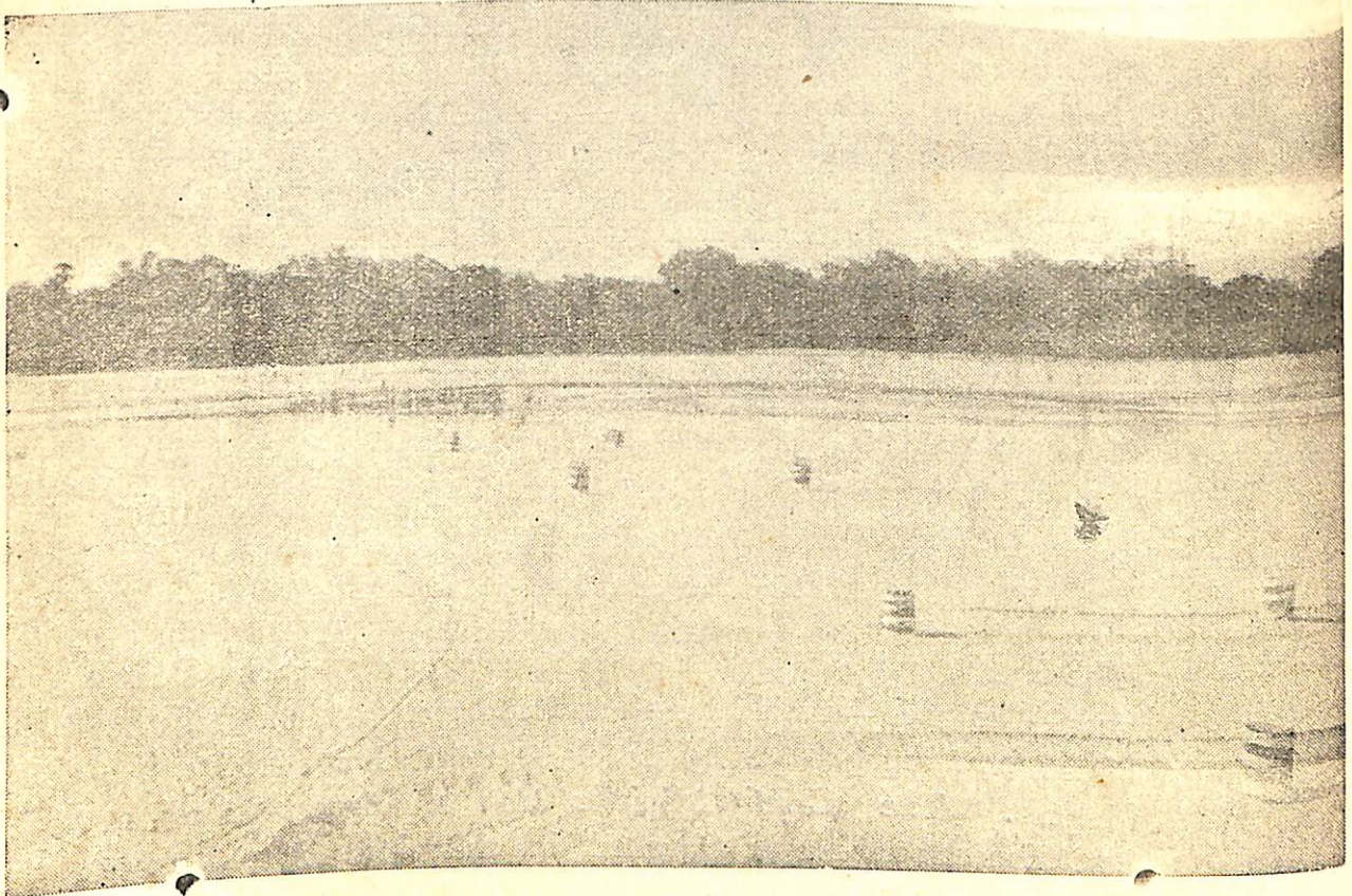
The demarcated site for the new Rushikulya bridge near Purushottampur
